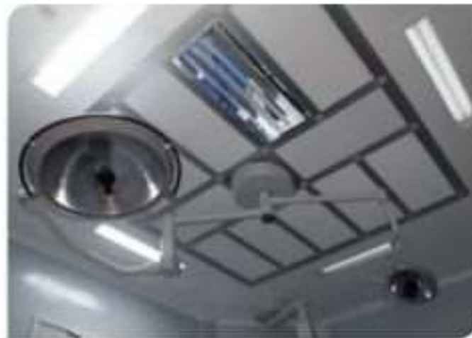
In Ceiling disinfection unit
